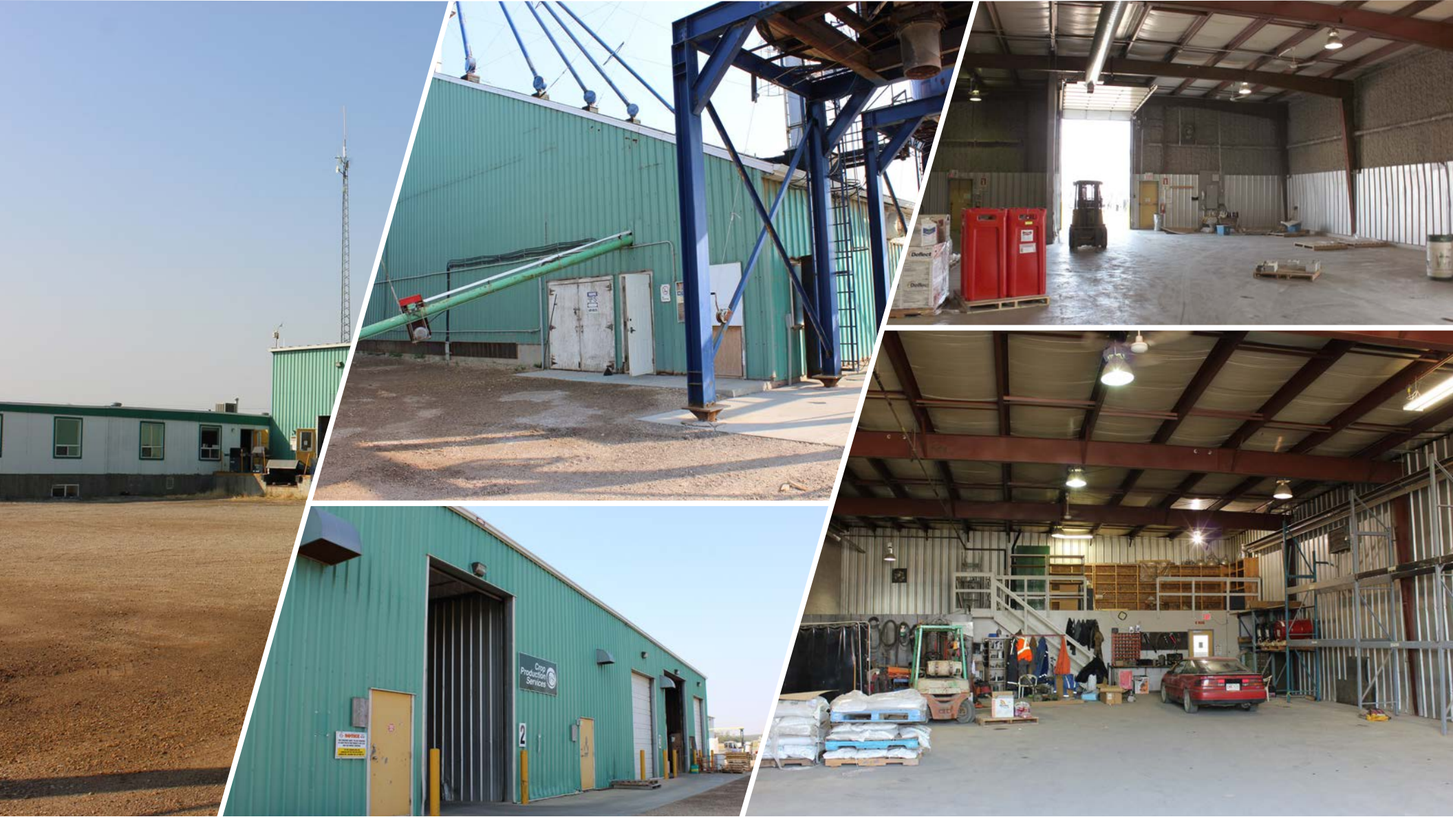
CLOCKWISE FROM TOP LEFT: Office Building // Bulk Plant Area // Interior Shop Area // Interior Shop Area // Shop Loading Area
